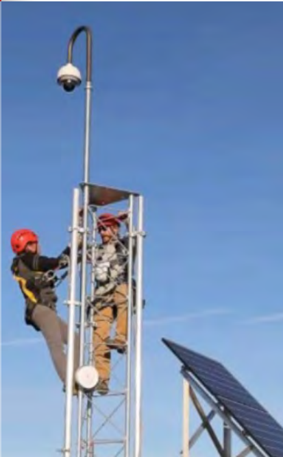
Fire Camera Installation
