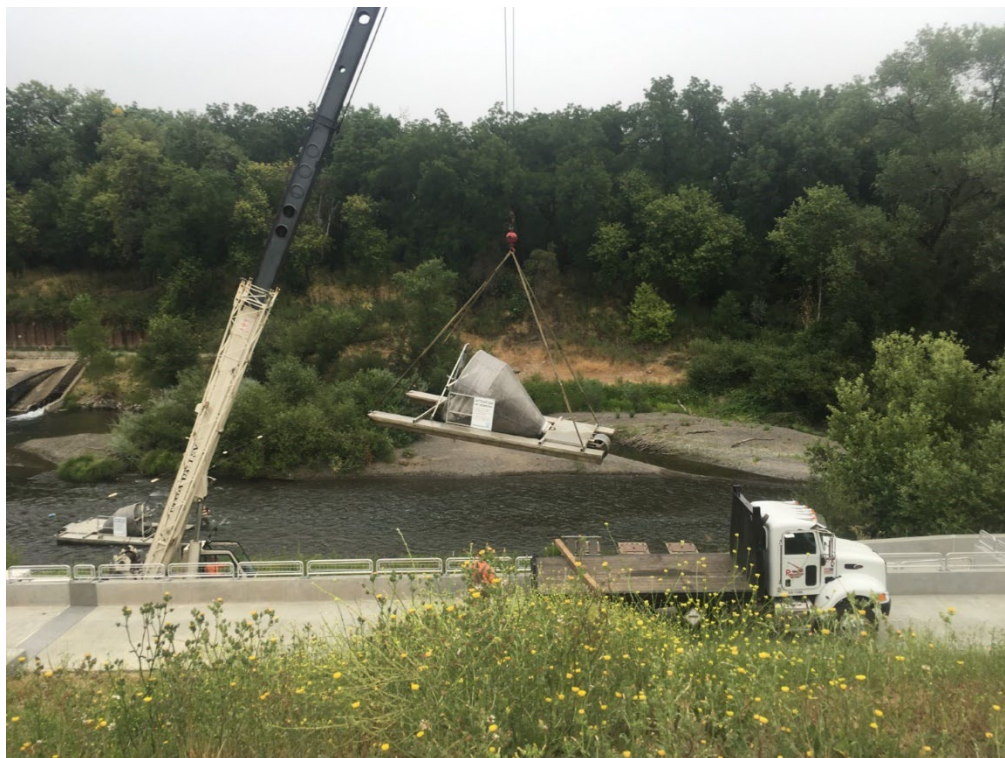
Heavy fish trap removal with crane part 2
