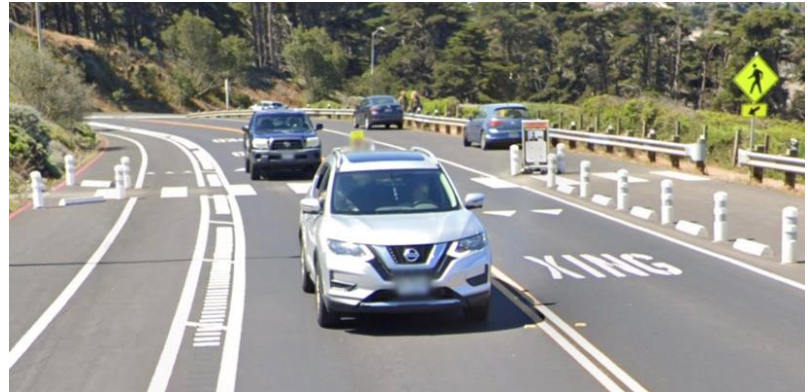
Example of a street with narrow lanes and buffer treatments to reduce speeds.
