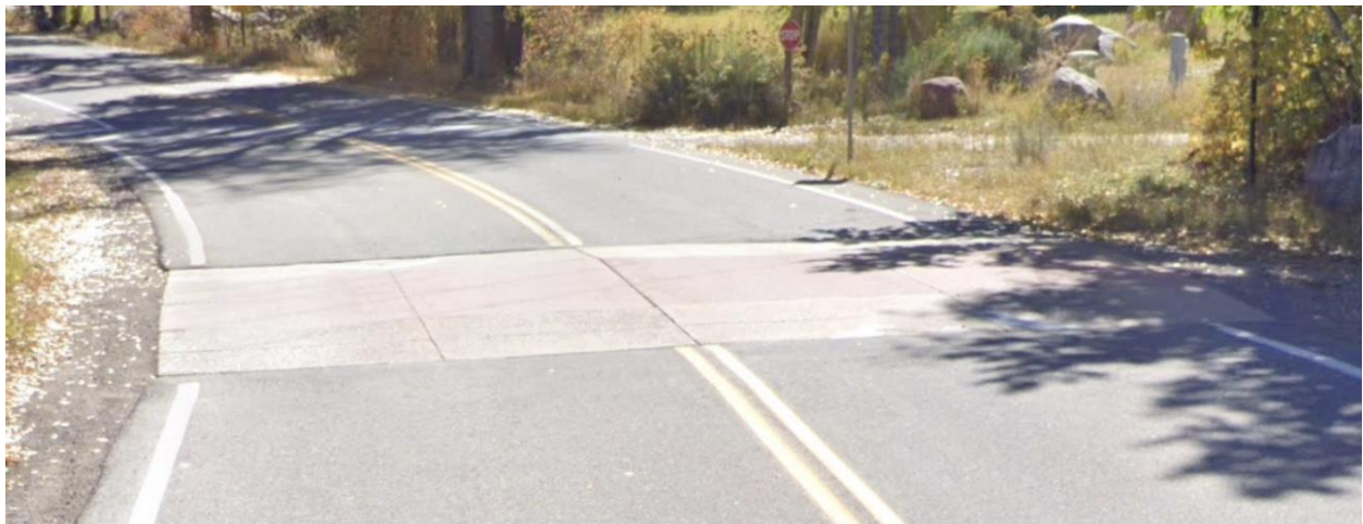
Example of a Speed Table on a 2-lane rural road near Aspen, Colorado
