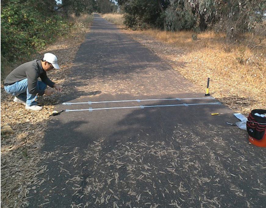
Installing tube counters
