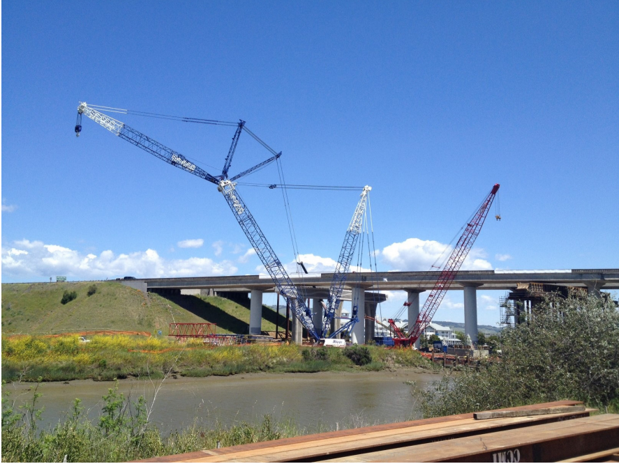
Construction at Petaluma River Bridge
