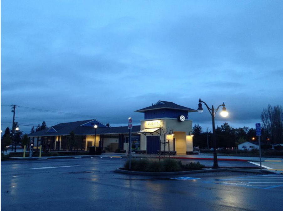
Cotati Train Depot - photo courtesy of Jake Mackenzie
